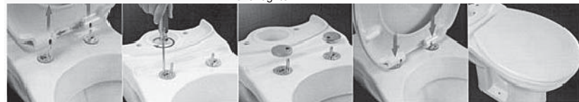
5) Lift the seat cover by pressing two pushbuttons. 6) Tighten the screws. 7) Place covering caps on the hinges. 8) Insert the seat cover 9) Finished onto the toilet.
